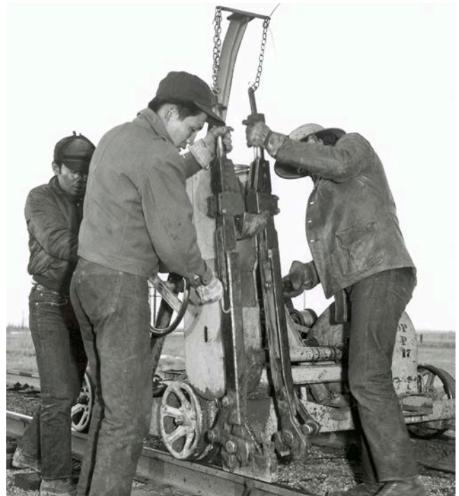
Navajo Trackmen work together to make the rails even. Photo from Union Pacific Museum.
